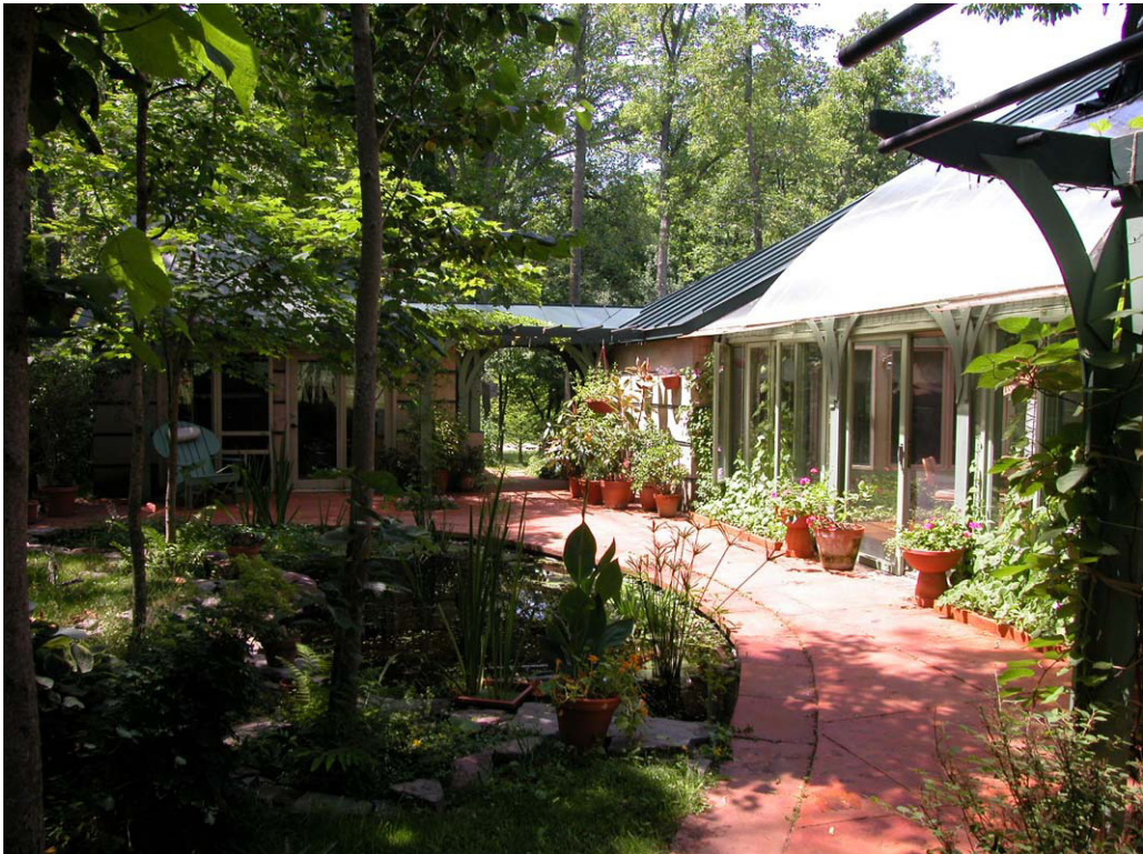
No part of this document may be reproduced without the consent of the office of GroundSwell Architects. © 2015 GroundSwell Architects
